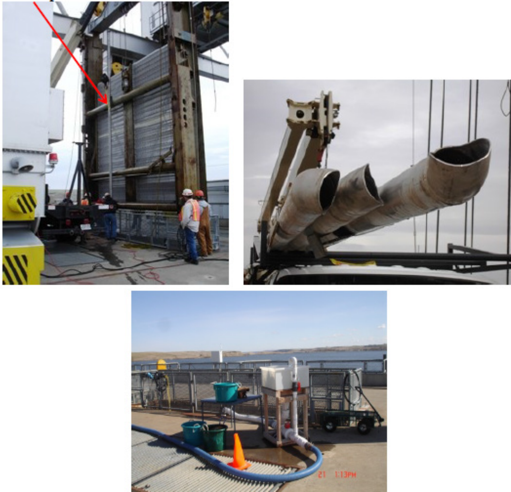
Figure 2: Planned fish release pipes design and method of attachment to traveling fish screen frame (top left photo) 30 inches off-center toward the north. Normandeau recommends that pipe design and installation (provided by Corp) follow that utilized previously in the 2007 study. The exit end of release pipes were curved (top right photo) and oriented in a downstream direction when installed. Normandeau will provide the same type of induction system and release hoses (bottom photo) used in 2007.
